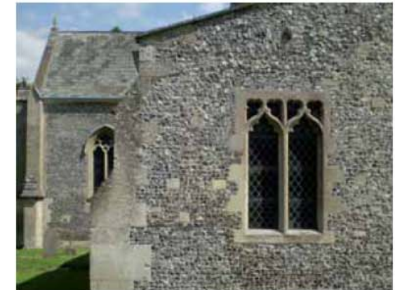
St Mary's Church, Great Bedwyn is built of rough field flints with limestone dressings for windows, buttresses and basal plinth.
