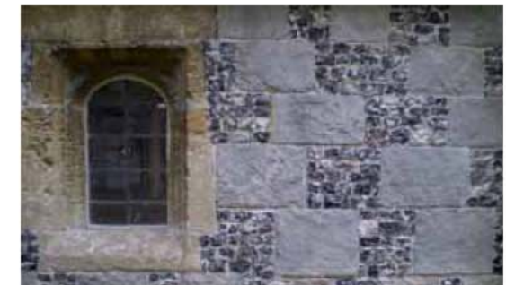
St James' Church, Avebury. Knapped flint and cut sarsen chequerwork with limestone window frame.
