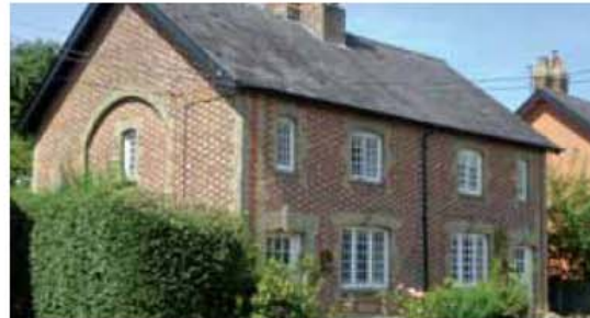
Combined red and grey patterned brickwork, Great Bedwyn.
