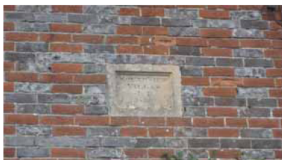
Glazed and unglazed patterned brickwork, South View Villas, 1896, Kintbury.
