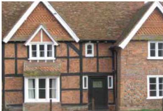
Timber-framed house with elaborate chevron-patterned brick infill and tile hung gable, Chilton House, Chilton.
