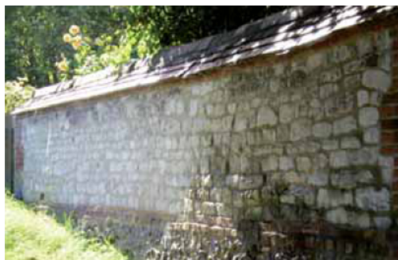
Chalk clunch wall with a protective tile capping and stone base to stop rising damp, Blewbury.
