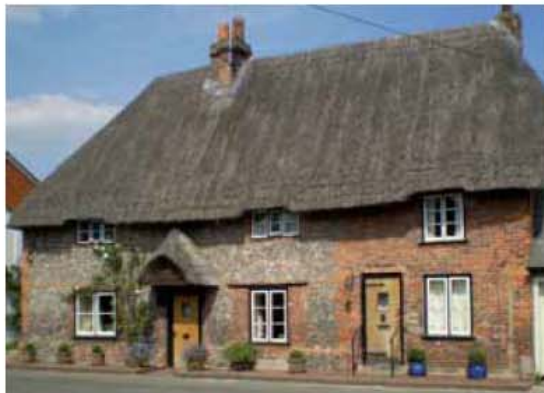
The Old School House, Hurstbourne Tarrant with thatched roof, rough flint walls and brick framing. The use of all brick in the the Old Bakery next door may indicate that this is a later extension, built at a time when brick had become less expensive.
