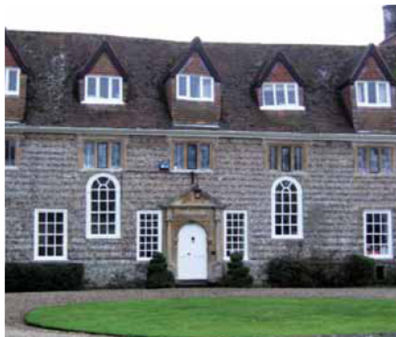
Alternating courses of cut sarsen and flints. Manor farm at Ogbourne Maizey.
