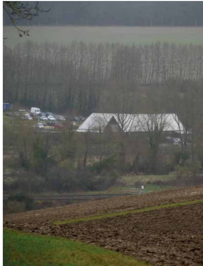
Highly reflective roofing material
