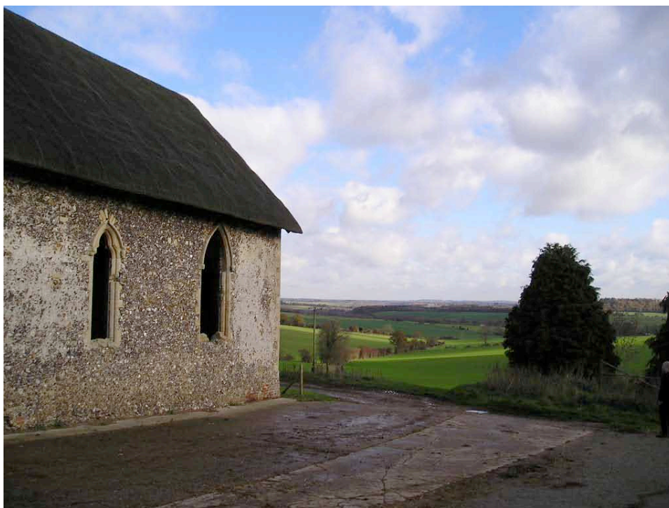
Churches like this one at Chisbury of are often built of flint as it is more durable than chalk.
