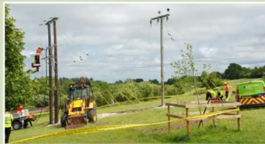
Cables being moved underground at Hungerford Common
