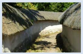
Lime-washed cob walls at Blewbury, protected from the weather by a thatch capping and rising damp by a stone base.
