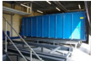
Fuel reception by 3 'hook lift' bins (2,600 tonnes per year of unseasoned woodchips sourced from woods managed on the Isle of Wight)
