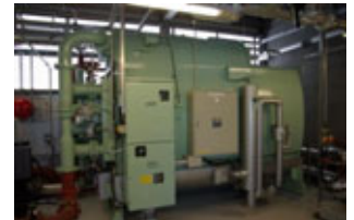
Heat is also used through an 'adsorption' chiller to deliver the cooling needs of the store in the summer but can be sold to neighbours in the winter.
