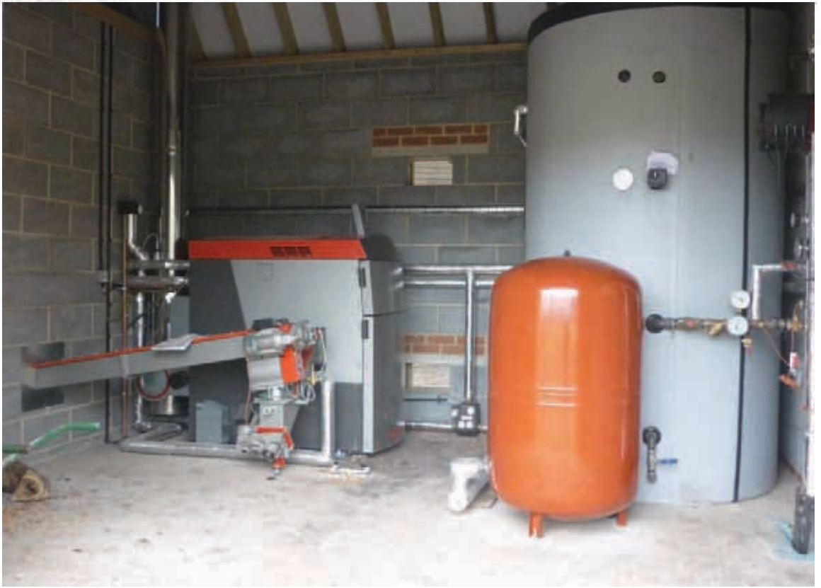
Woodfuel boiler and buffer store. The new woodfuel boiler is on the left, and the 3,000 litre buffer store is on the right. The silver box coming through the wall on the left is from the woodchip store and houses the screw conveyor which automatically feeds the boiler with woodchip.
