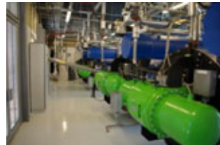
Woodchips are fed to updraft gasifiers, gas is burnt and heat is used in 4 Stirling engines to create electricity
