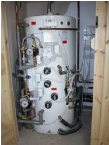
Domestic accumulator drawing heat from a wood burning stove and solar thermal array, with electric emersion coils for frost protection when owner is away in winter
