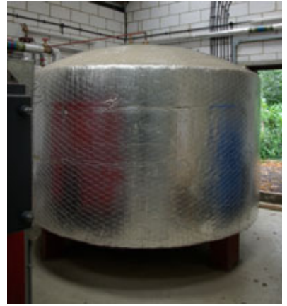
'Large' accumulator working with a 250kW boiler to heat a former stately home (or 'schloss')
