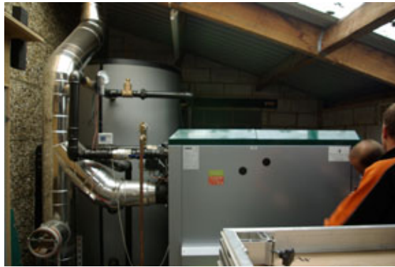
Accumulator (left rear) linked to a 100kW boiler (right centre) to provide heat for a community building
