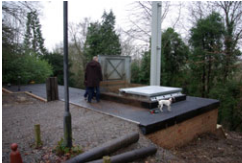
Access doors for 'tipping' woodchips into bunker are sited in the centre of the bunker.
