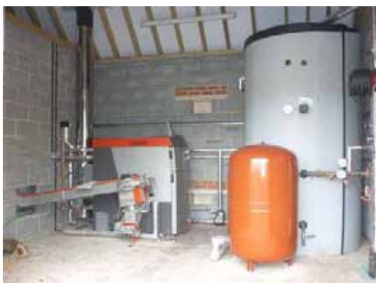
The 60kW woodchip boiler installed at Manor Farm, Hampstead Norreys is shown on the left, with the 3,000 litre buffer tank which stores the heated water on the right. ©Meg Chambers
