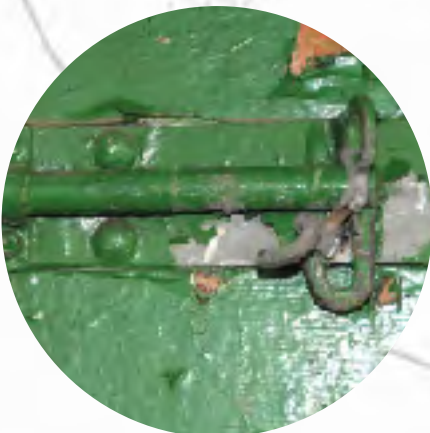
Vandalised garage door bolt
